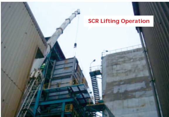
An air pollution control prevention equipment was added in the Shulin plant
