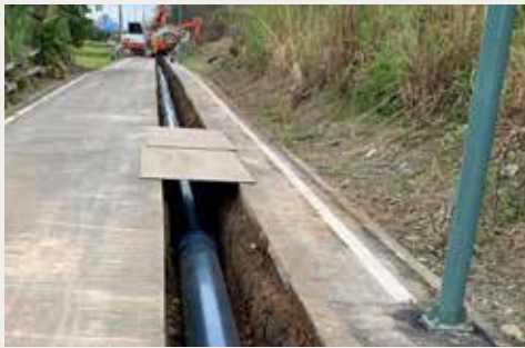
Tap water piping projects
