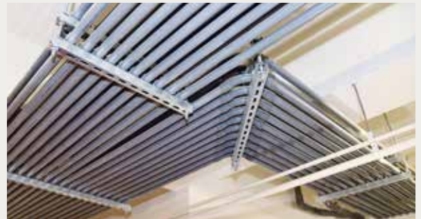
建築工程 Architectural engineering
