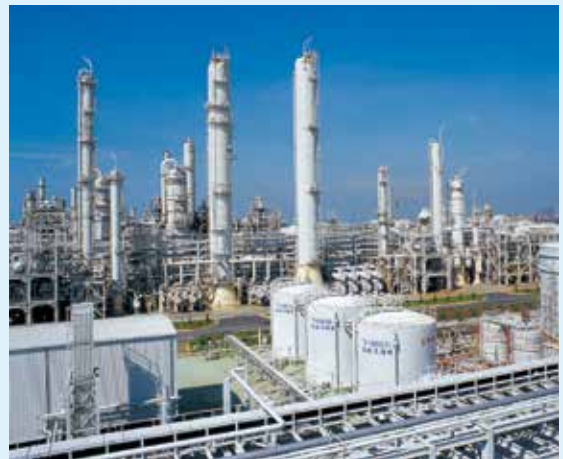
工廠排水配管 Petrochemical plant
