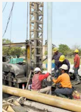
鑿井工程 Well drilling engineering
