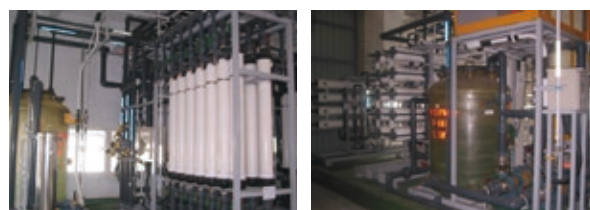
Wastewater recycling technology – Reverse Osmosis (RO) & Ultra Filtration (UF) equipment
