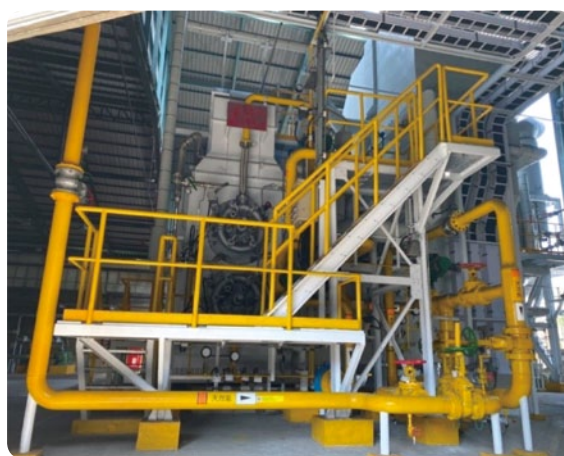
50 tons gas-fired boiler
