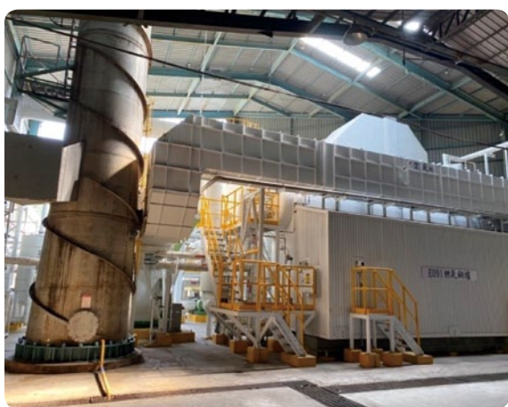
Appearance of gas-fired boilers in Shulin site
